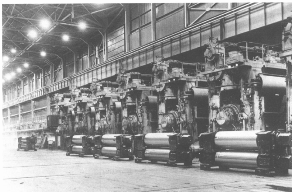
Fig. 20 Finishing stands of a 2130 mm (84 in.) hot strip mill. Courtesy of Mesta Machine Company
