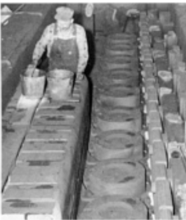
Fig. 6 Dry sand pit mold for stationary diesel engine.
