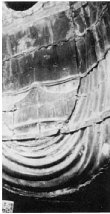
Fig. 13 View of the interior of the Kamakura Buddha showing the interlocking joints between the casts.
