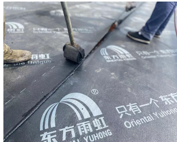
卷材搭接处采用辊压挤浆
