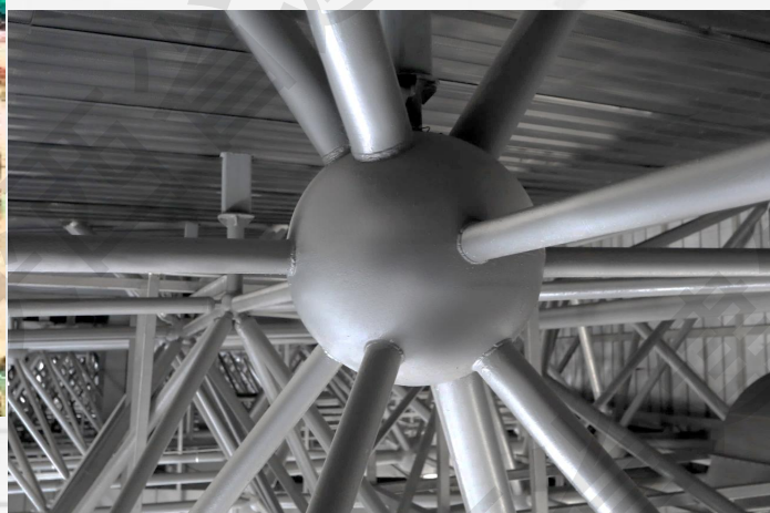
焊接球焊缝饱满
