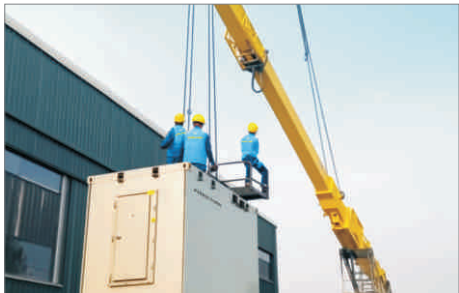
设备运输至安装基础位 Transporting the equipment to the installation base
